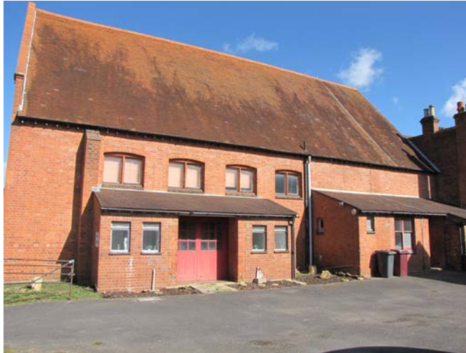
Rear elevation of church
