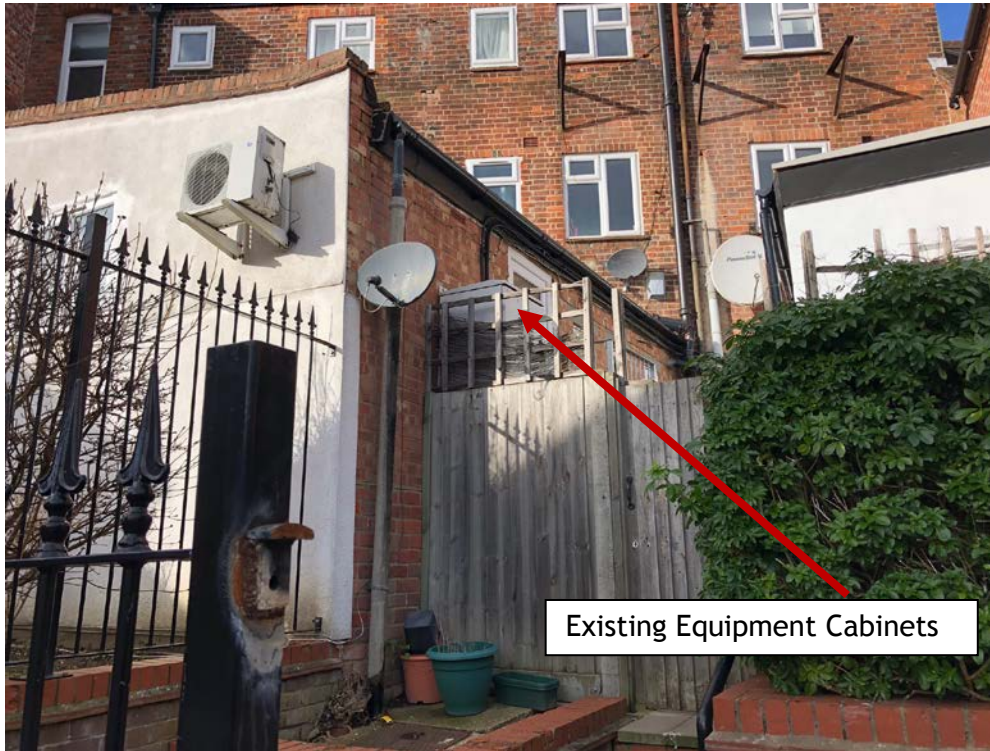
View of rear of building
